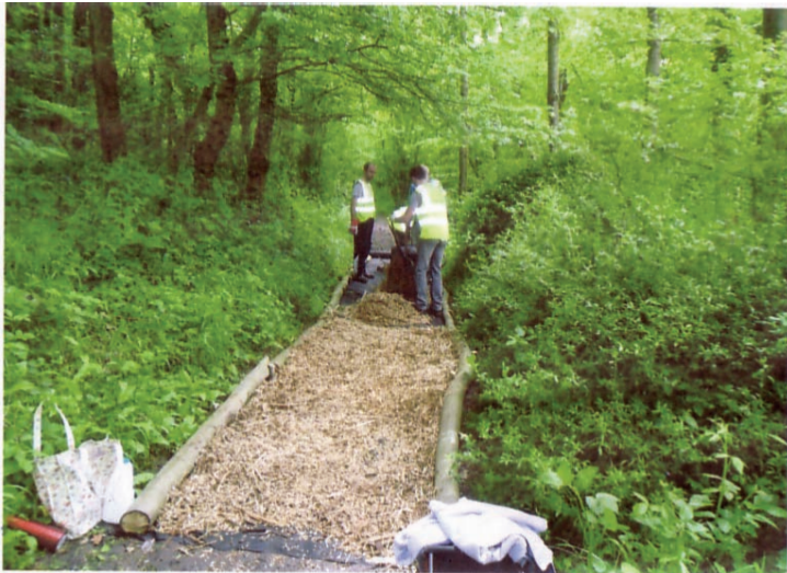
Friends of Beacon Wood progressing the footpath
